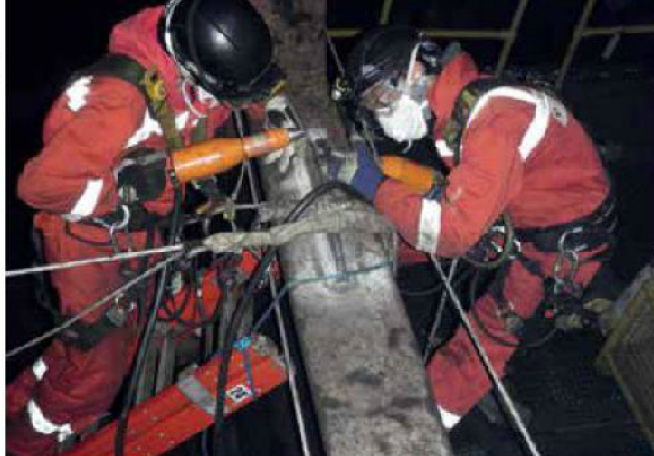
LETS Global Ultrasonic Peening Technicians working on the FPSO Schieballion
